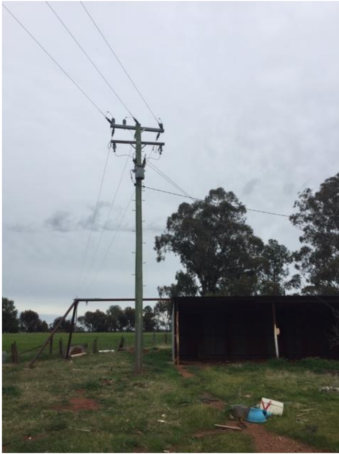
Existing power pole to be removed as part of subdivision
