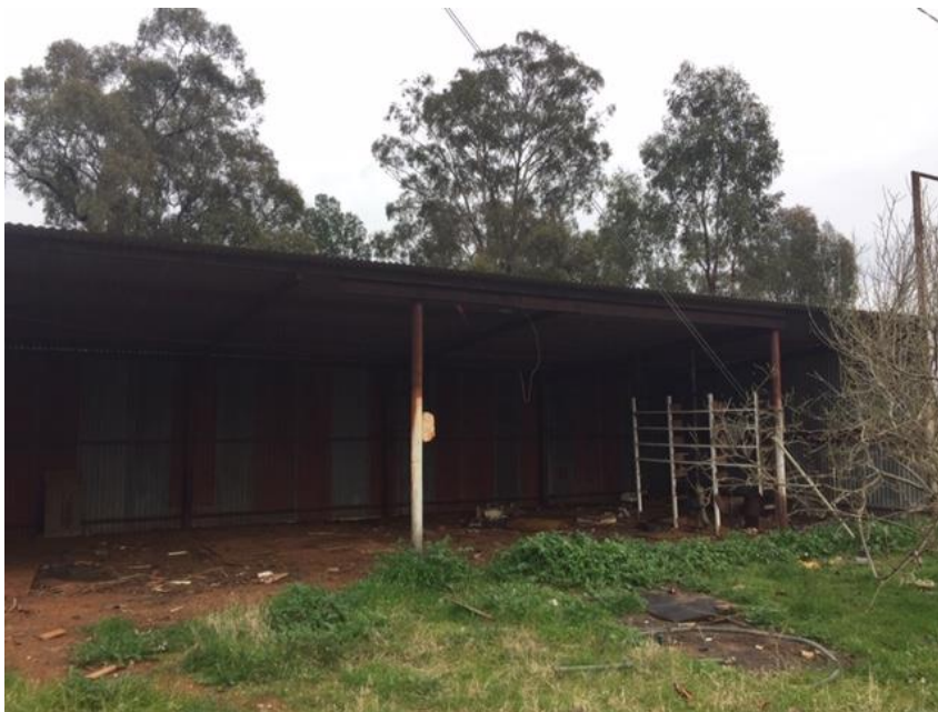
Photo 2: Shed located on Lot 1112
