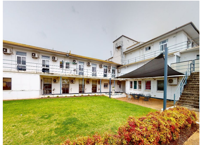
Picture 4 Back of Main Building (Northern side) behind Consultation Rooms.
