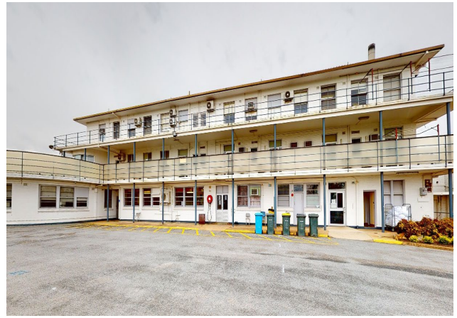
Picture 2 Back of Main Hospital Building.
