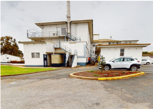
Picture 1 West side of the Main Hospital Building and Front of Boiler and Waste Room
