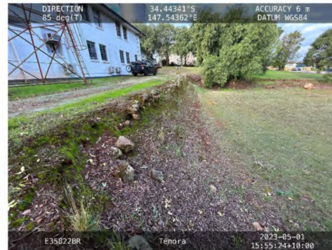
Photograph 12: Evidence of cut/fill
