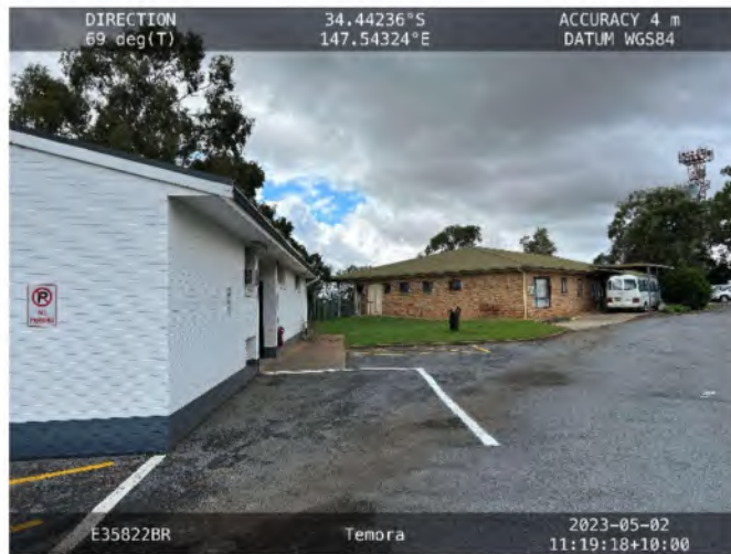
Photograph 3: Maintenance building and Day centre building
