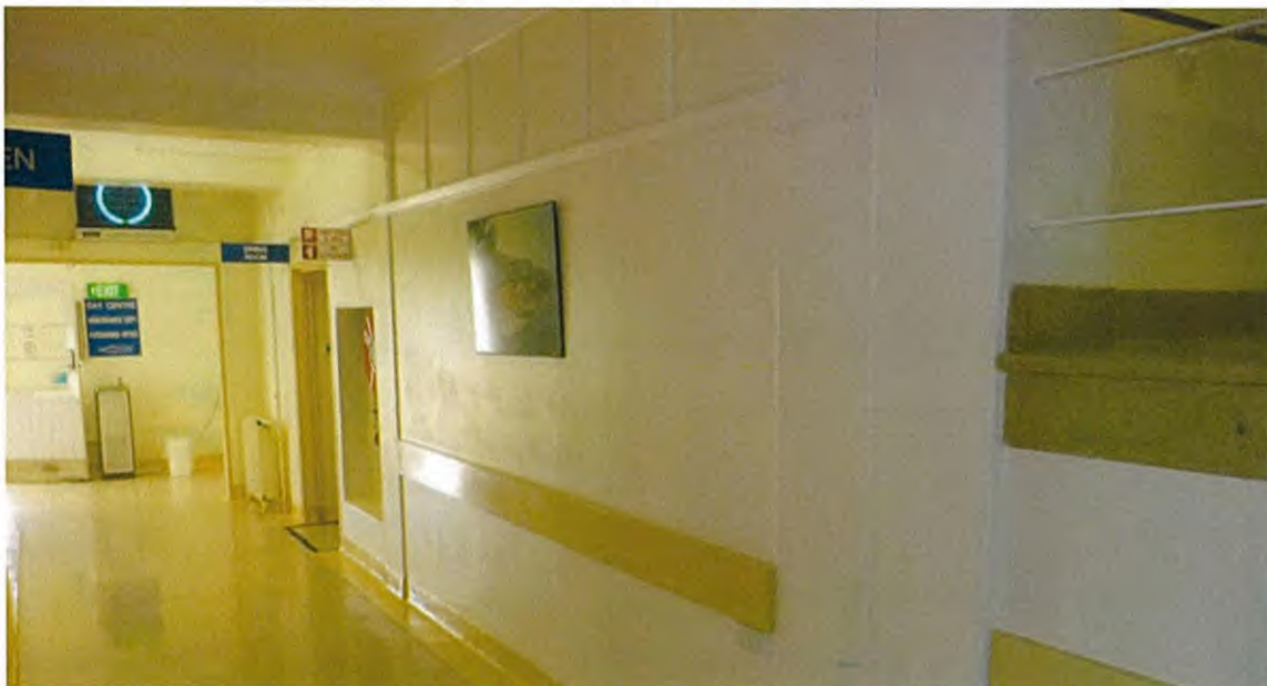
PHOTO: Internal corridor showing location of new lift.
