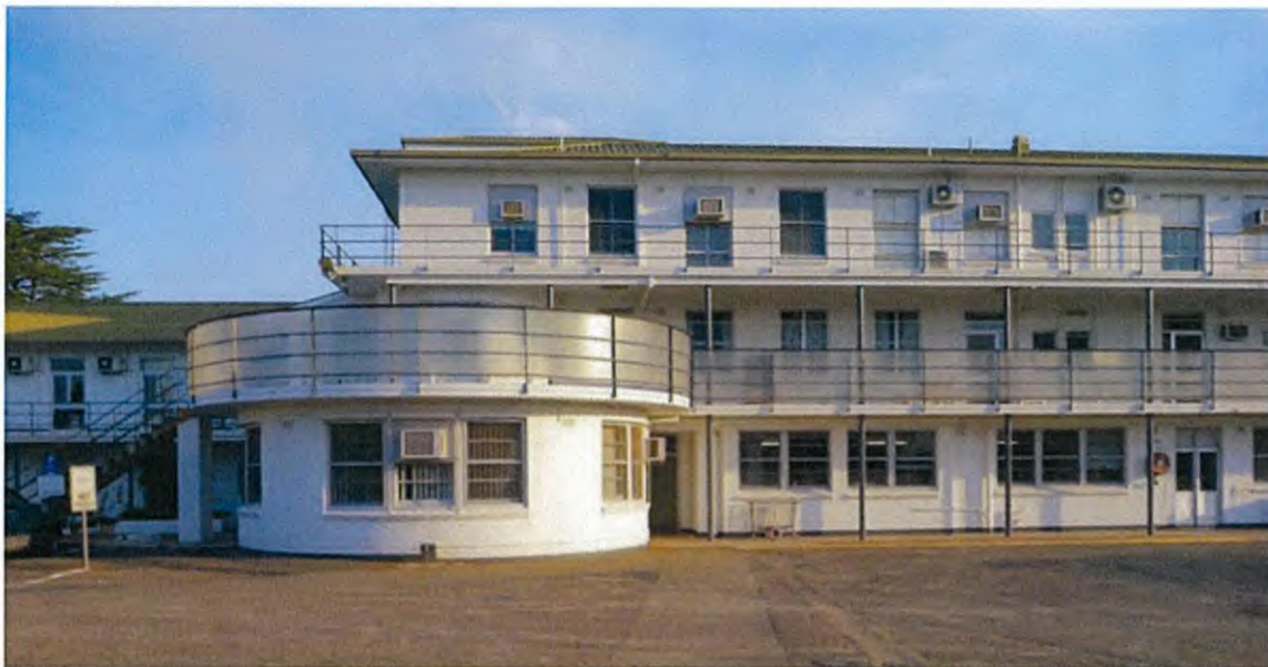
PHOTO: Exterior of Temora Hospital showing vicinity of new lift.
