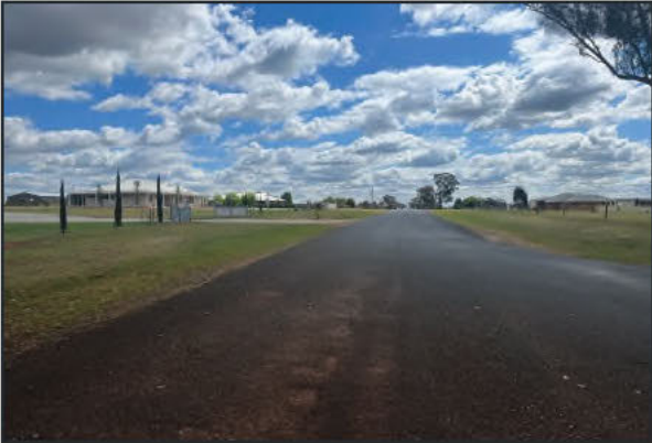
EVATT STREET LOOKING WEST
