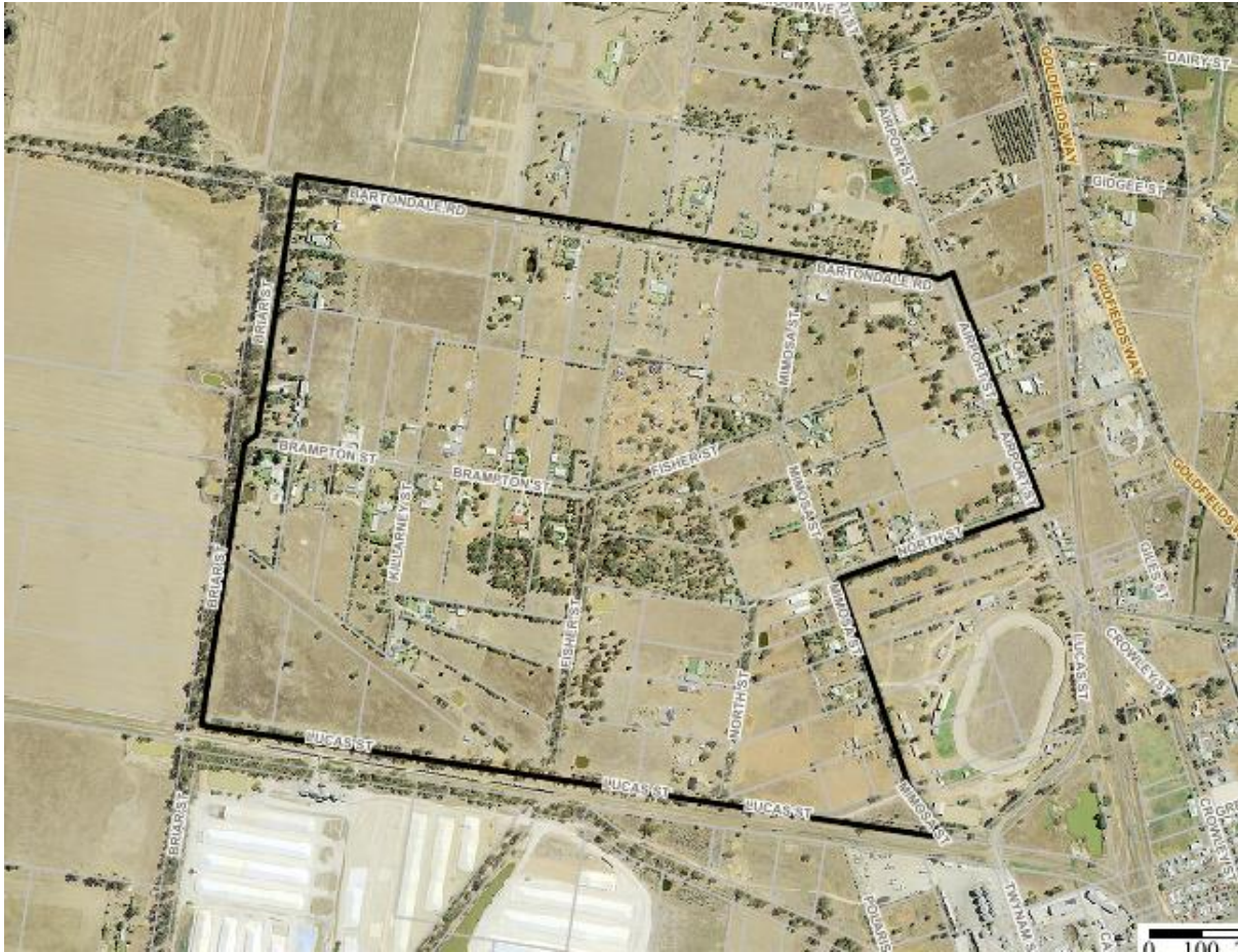
Figure 18: Existing large lot residential zoned land located on the western fringe of Temora, adjoining Temora Airport to the north
