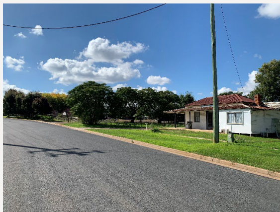
Figure 32 – Site 1 view of existing dwelling contained on Lot 2.
