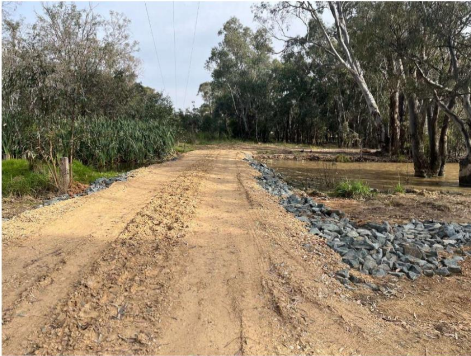
Photo 1: New walking path approach to bridge site
