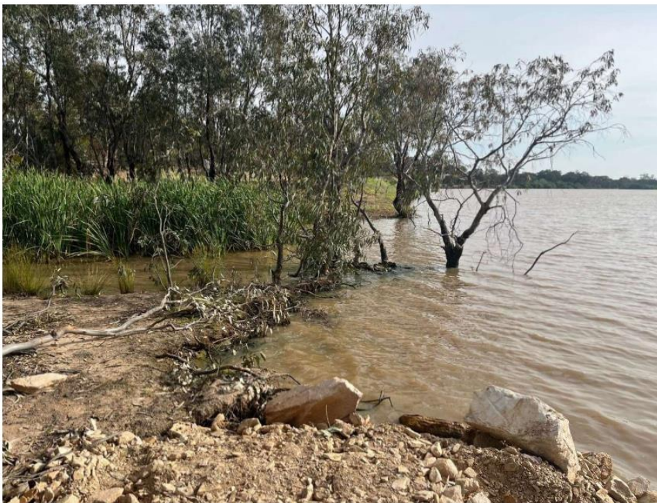
Photo 3: Site for bridge installation, noting high water level at this site
