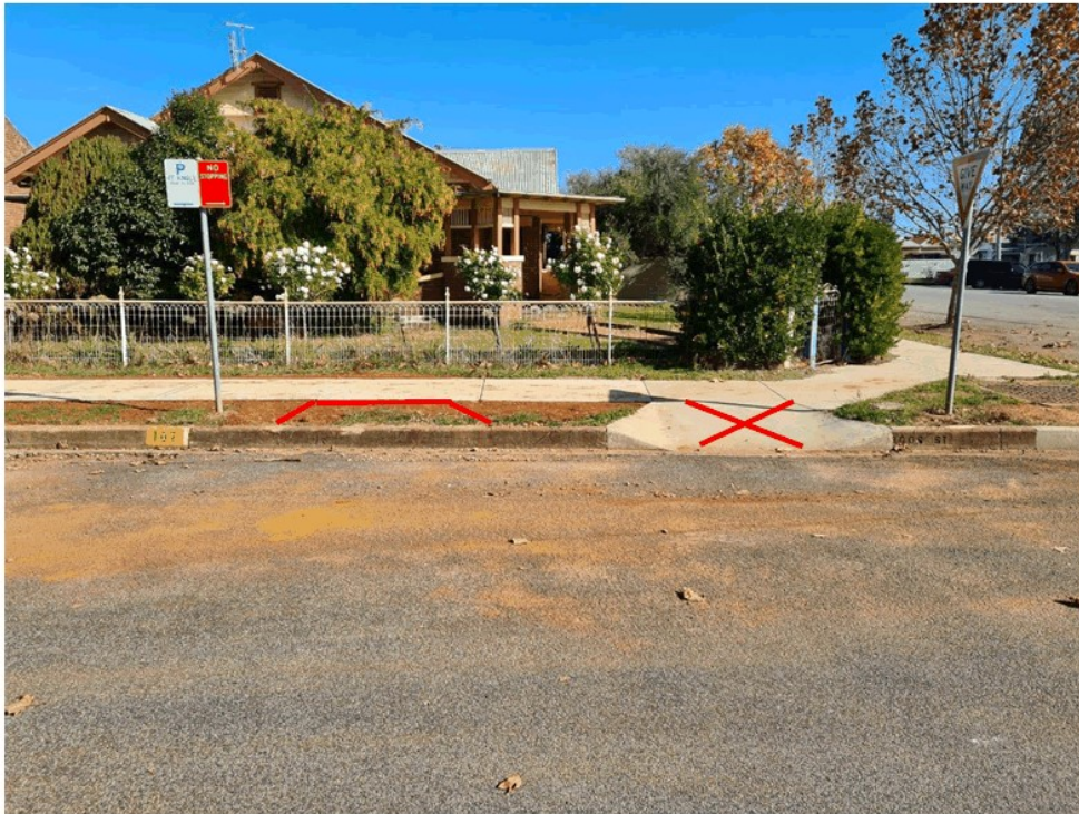
Image C: Proposed new kerb ramp location Western Side and remove existing kerb ramp
