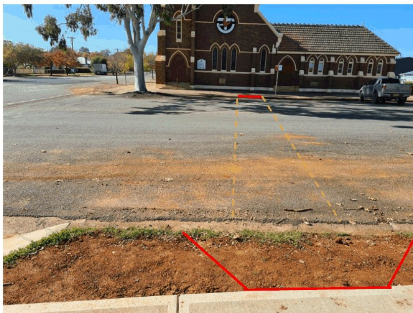
Image D: Proposed new alignment for both new kerb ramps on each side of Deboos Street (In conjunction with removing both current kerb ramps)
