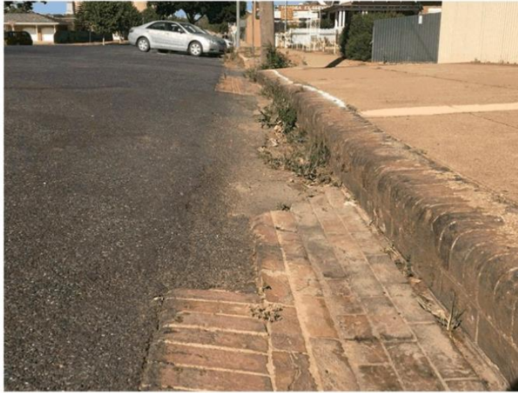
Photo 5 – Kerb defect
