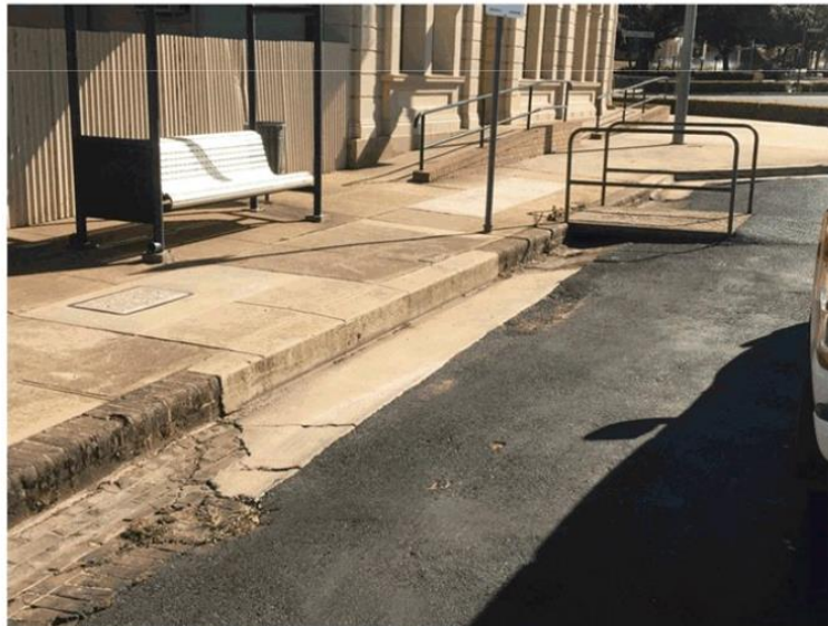
Photo 4 – Kerb defect
